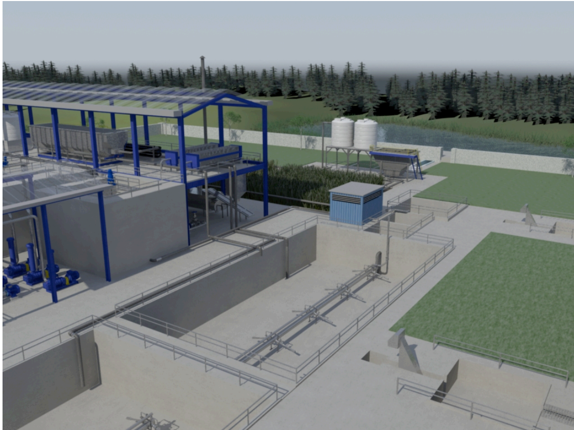
Picture 2: Primary effluent treatment plant with screening, balancing, sulphide oxidation and DAF
