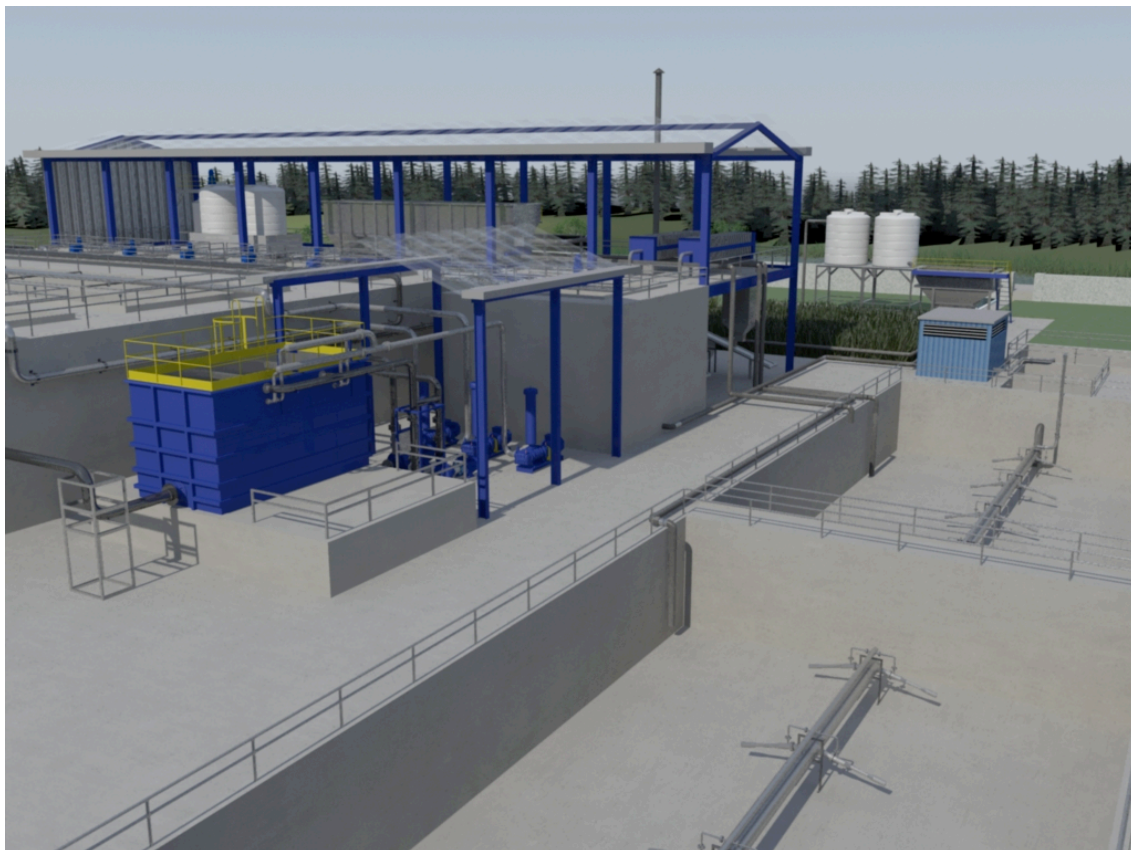
Picture 3: Biological effluent treatment plant with anoxic and aerobic biological MBR treatment
